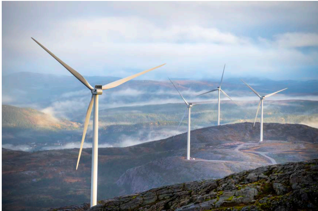
Åfjord Fosen 20201013. When Storheia wind farm was transferred to ordinary operation in February 2020, it became Norway's largest wind farm with 80 turbines. © Heiko Junge / NTB
